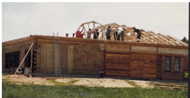
Volunteers erecting the hip roof on the Jackson Quartermaster building.
